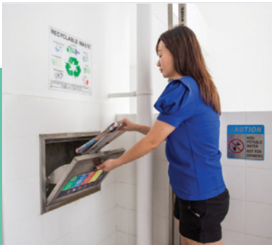
SEPARATE CHUTES FOR RECYCLABLE WASTE
